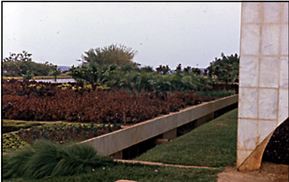
Parking garage, Brazil
