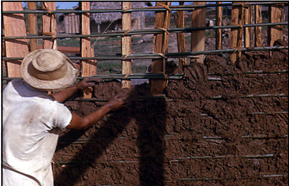
House Construction, Ze-Doca
