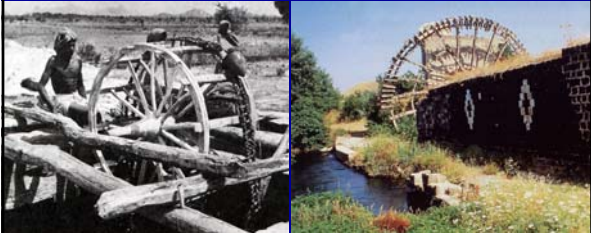
A Persian water wheel powered by a man's legs
